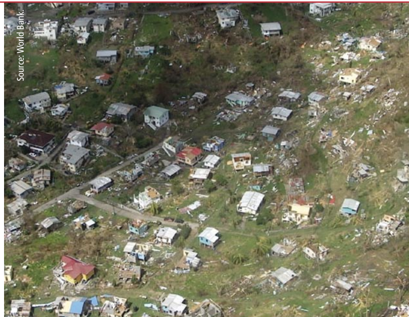
Close to 90 per cent of houses on the Island of Grenada were affected by Hurricane Ivan.
